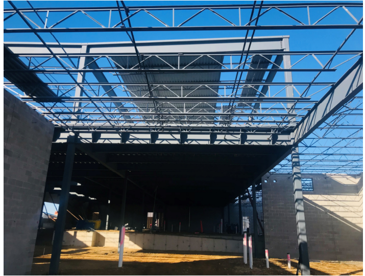
Steel Beams, Joist, Decking & Detailing in the Administration Area
