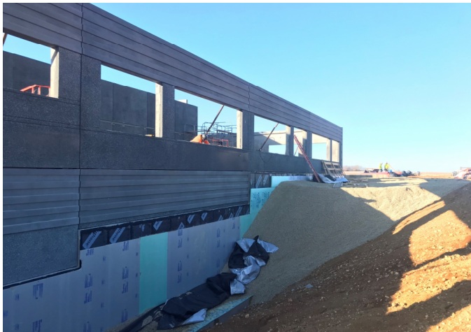
Backfilling, East Side of Gymnasium Wall
