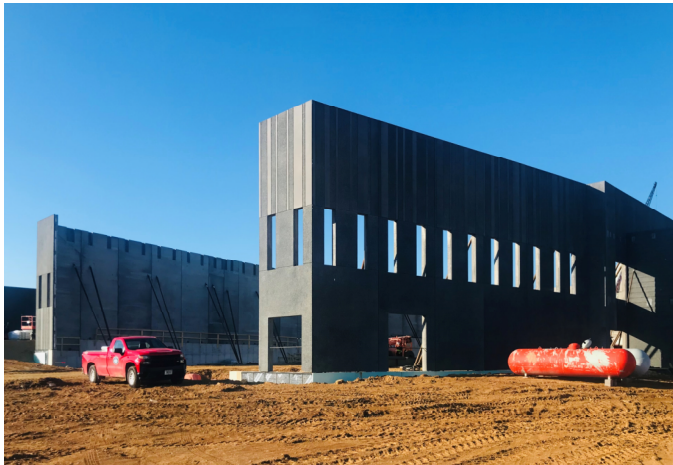
Precast Wall Paneling by the Gymnasium
